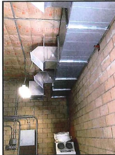
Installed ceiling insulation and AC air ducting
